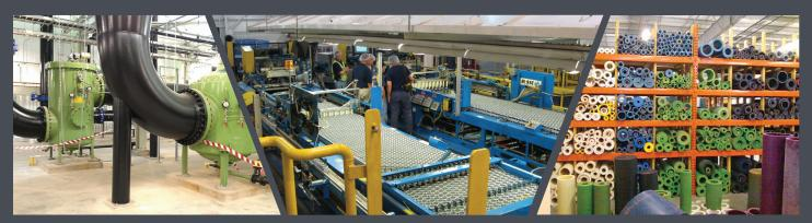
1: Engineering and design of an overall water recycle system for this seamless steel pipe manufacturer in Youngstown, Ohio, included these final strainers to supply clean water for contact and non-contact cooling.
