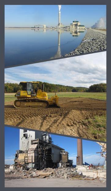
1: Water quality and quantity were analyzed to adjust the original water balance at this Illinois coal-fired power plant designed for zero liquid discharge. 2: Field testing of 15 capping scenarios and constructability of the most promising alternatives for a 965acre CCR disposal impoundment in Pennsylvania. 3: Environmental investigation, mitigation, and demolition activities for numerous multiunit boiler houses, ancillary structures, and equipment at six retired generation stations in Ohio
