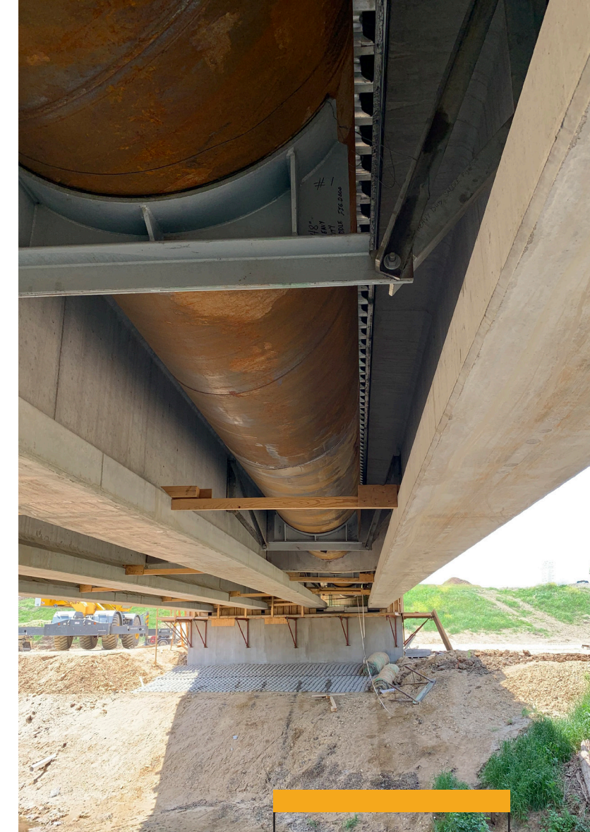
CEC's design integrated and embedded a carrier pipe for a landfill gas pipeline.
