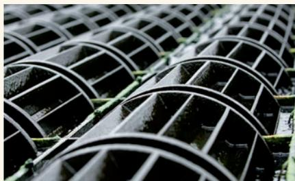
*Algaewheels grow algae in a controlled environment. In turn, algae produce oxygen, which bacteria in the system use to convert wastewater organics into carbon dioxide.*
