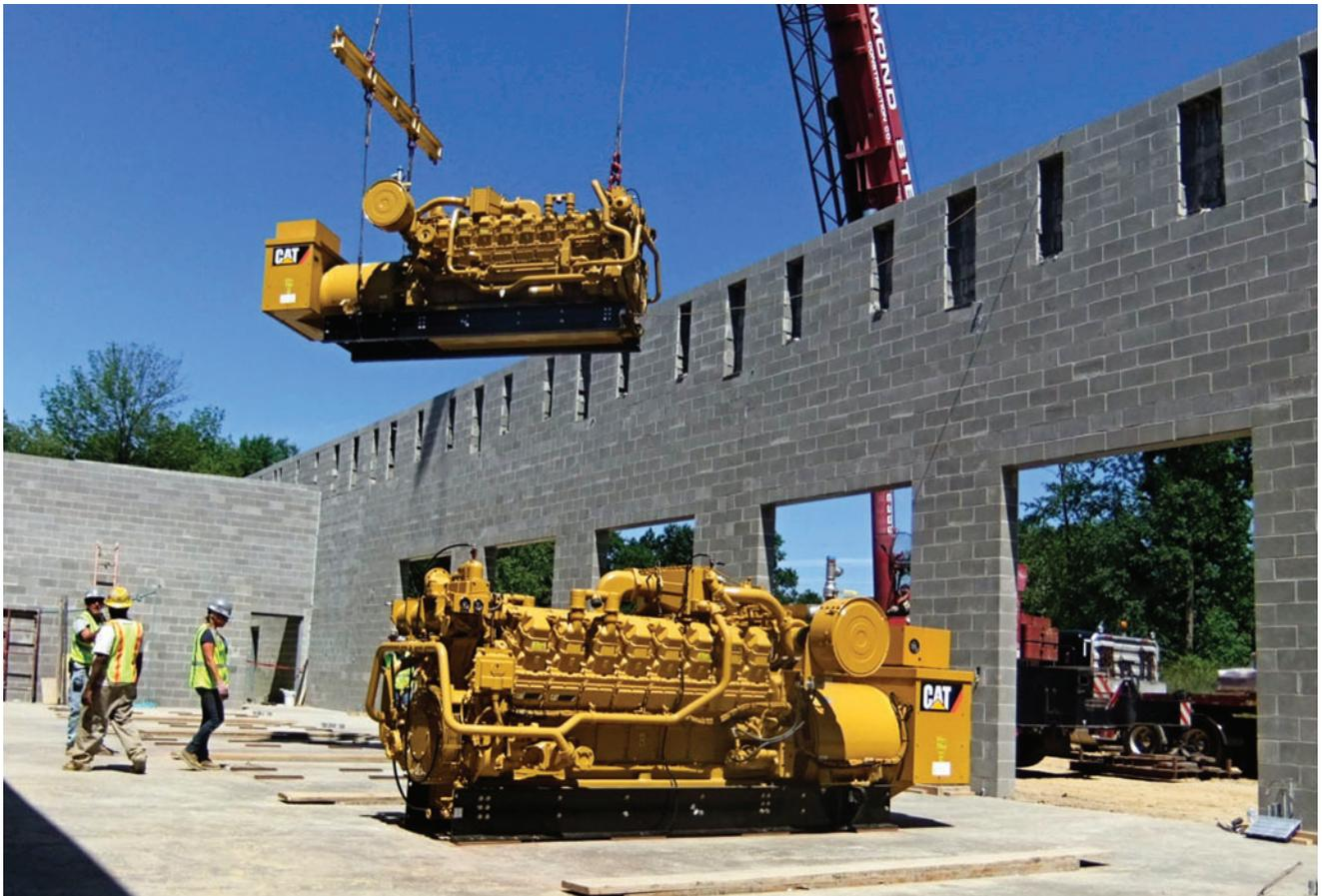
These enormous CAT engines will utilize landfill gas to create electricity at a new Landfill Gas to Electric plant.
