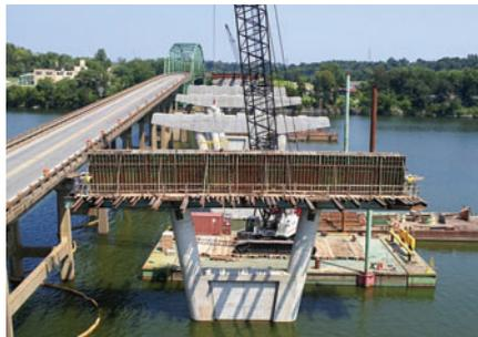
*The new bridge is a composite deck slab bridge with precast, prestressed 72" bulb-tee beams and welded steel girders. It will have four lanes, eight piers, and be 1,616 feet long.*
